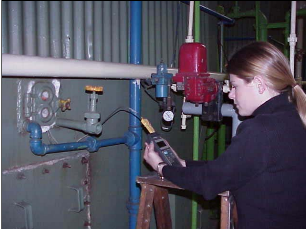
Fig. 10, Furnace temperature measurement system
